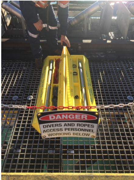
Rope access personnel trialling prototype Gridmesh Anchors
